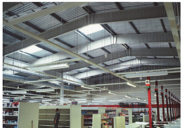
Fig. 2. Building structures of corrugated web girder
