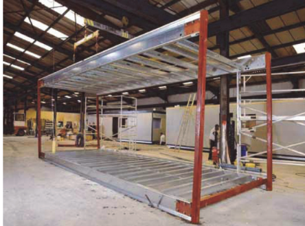
(b) With light steel floor joist (Kingspan)
