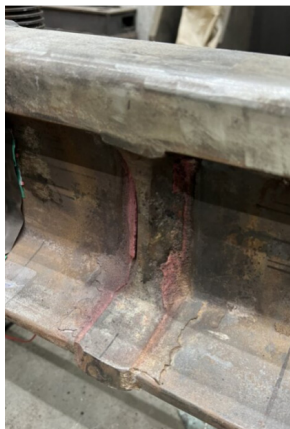
Fig. 7. Weld reinforcement thermite joint
