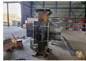
(c) Assemble the upper column and KG beam
