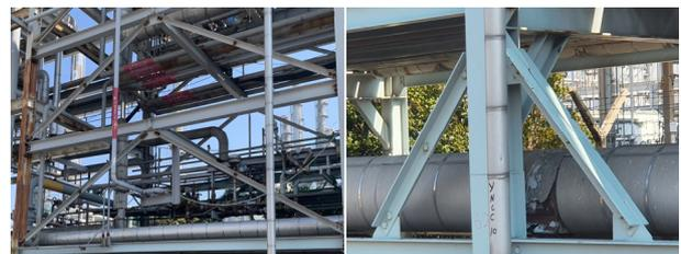
**Fig. 1.** General configuration of piperacks consisting of typical double angle bracing members, columns, and beams
