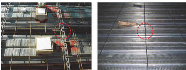
Fig. 2. Prevent flaring of the upper deck
