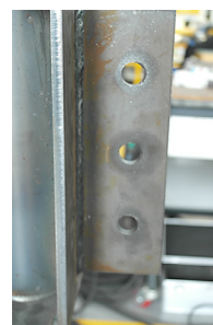
(c) Bearing deformation observed in bolt holes of beam
