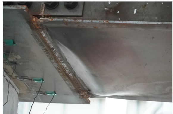
Fig. 11. Failure shape of HF-SRC-BM
