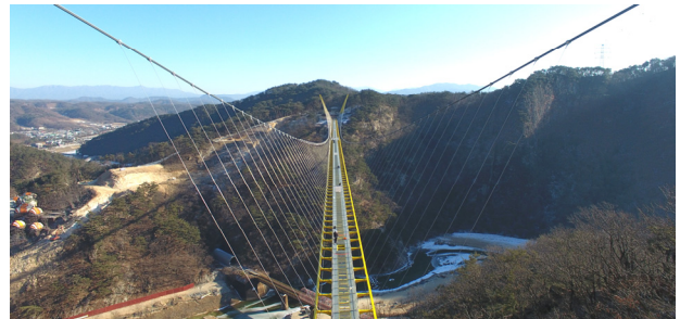
Fig. 21. Appearance of 3D cable system
