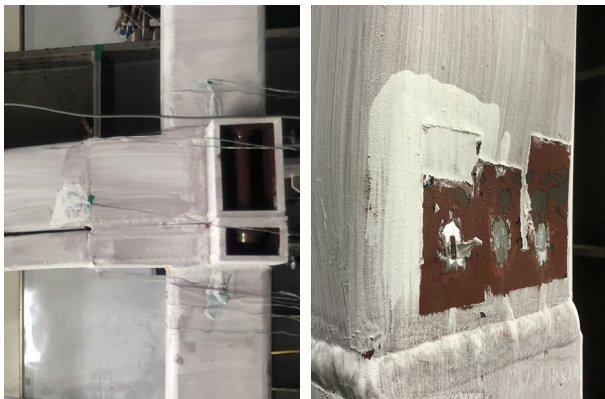
(a) Deformation at 4% drift (b) Buckling in ceiling beam at 4% drift
