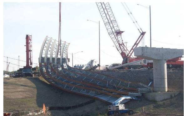
Fig. 1. Rollover due to lateral torsional buckling<sup>[7]</sup>
