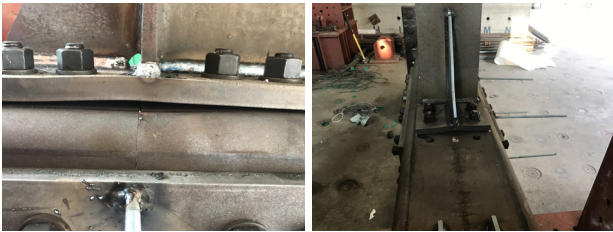
Fig. 9. Test specimen IP9 at the end of the test
