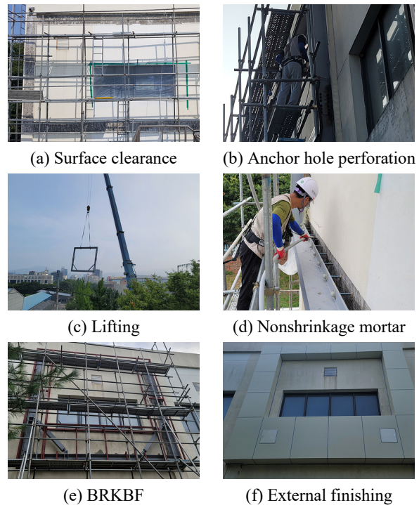
Fig. 3. Construction procedure of BRKBF method
