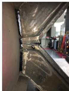
(b) T1 (crack in stiffener weld)
