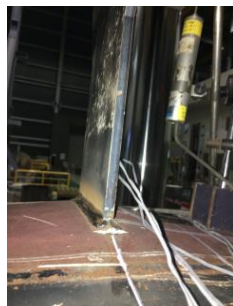
(a) N1 (out-of-plane buckling of the central plate)
