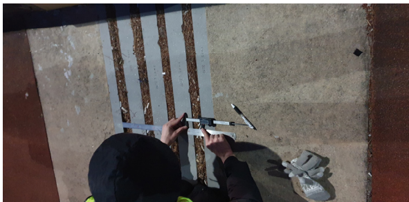
Fig. 4. View of the clearance measurement of the study bridge
