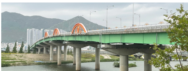
Fig. 1. Complete view of the study bridge
