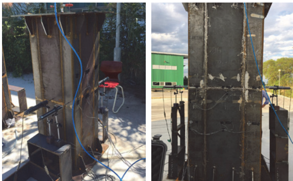
(b) Installing the measurement sensor
