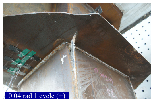
Fig. 10. Crack of column and external diaphragm (HF7-DC6-BB8)
