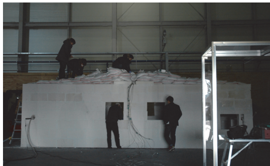
Fig. 11. Vertical static load applied using 400 sandbags (8 ton)
