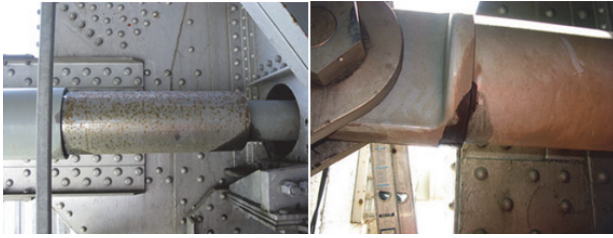
Fig. 1. Leaking in fluid damper [9]
