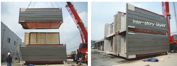
Fig. 2. Inter-story layer in modular building
