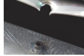
(a) Destroyed aspect (b) Tear panel
