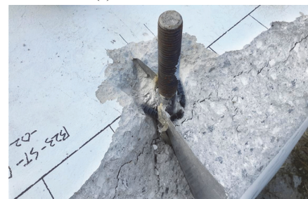
(b) rebar failure
