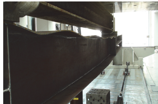
Fig. 1. Coupled buckling mode of plate girder
