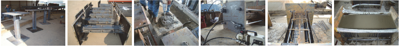
① Base column ② Installation of stud and anchorage ③ Concrete casting at base column ④ Pre-loading ⑤ Assembly of form ⑥ Encased concrete
