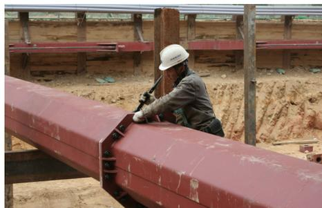
Fig. 2. Splice of OHS at mid point
