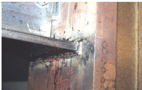
(b) Elimination of notch through flushing and grinding
