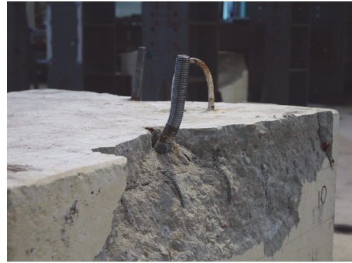
Fig. 16. Typical concrete fracture of stirrup reinforced anchor
