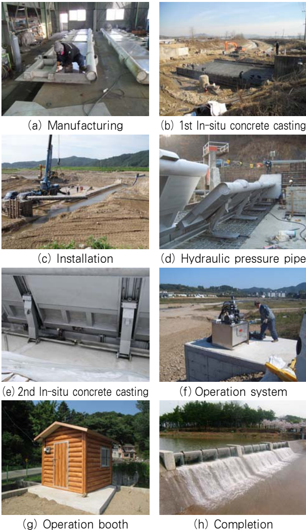
Fig. 6 Construction process of multistage overturning movable gate (6)
