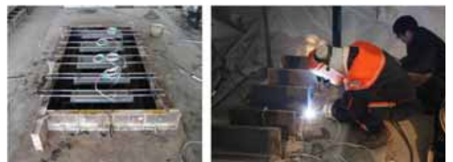
Fig. 2 Specimens before placing concrete and weld heat measurement
