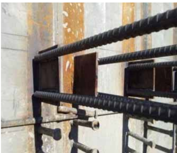
Fig. 4 Example of moment plate connection
