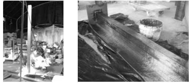
(a) Steel tube welding (b) FRP sheet retrofitting
