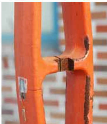
Fig. 20 Gap Part Corroded
