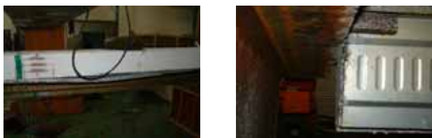
(a) Deck bonded failure (b) End slip
